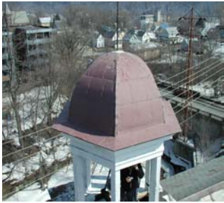
Cupola framing and trim repairs and a new bell deck are needed.
