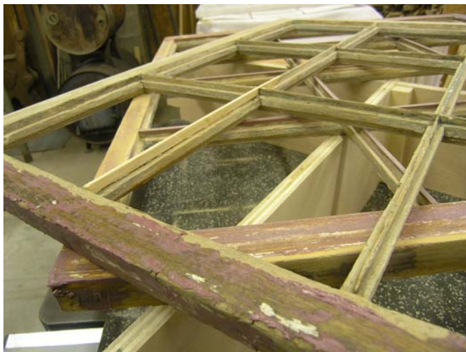
In the shop—window sash with glass carefully removed, paint dipped away, ready for wood and epoxy repairs.
