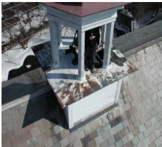
Cupola framing and trim repairs and a new bell deck are needed.
