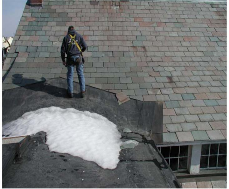
Slates no longer secured because of failing nails have slid down the roof and rest on the tower flashing. More lie to the right of the snow bank.
