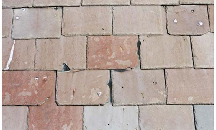
Popped nails have worn holes from the underside into and right through the slates above them. Nail holes and cracks have been unsuccessfully treated with sealant.
