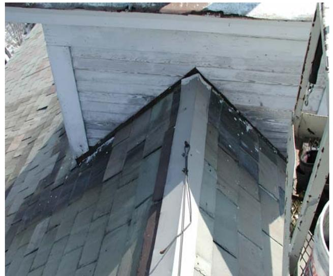
**S**heathing. In 1846 the Armory roof consisted of wood shingles over board sheathing. Ca 1880 when the slate was installed, two layers of wood shingles were left in place underneath. Moisture increasingly held in this relatively thick, now spongy underlayer prevents the nails from holding the slates firmly and prevents the slates from being evenly supported. Many slates have slipped.
