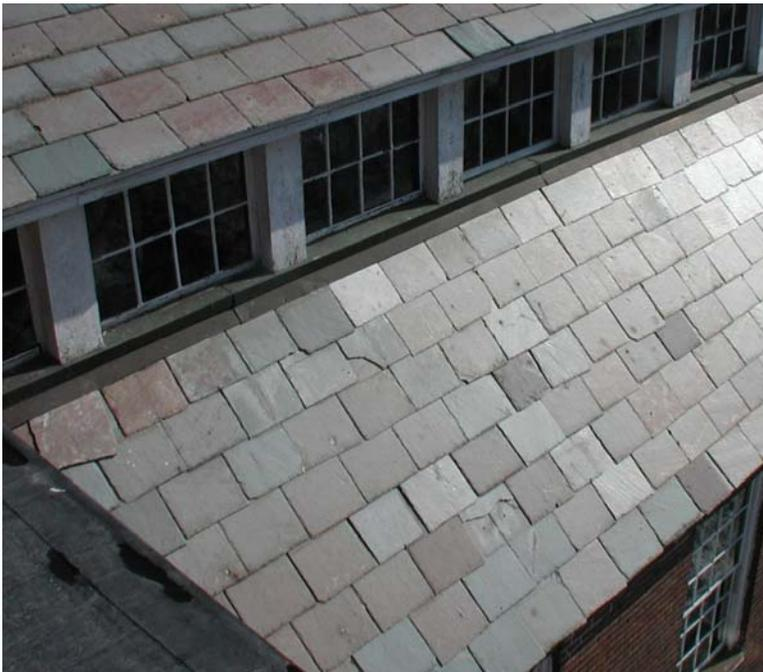
Weathered, loose, cracked and slipped slates.
