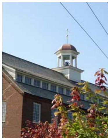
**Cupola** An important and original architectural feature, the bell signified the change from artisan process to the factory system as it called shift workers to the Armory. This timber framed, hexagonally-columned structure has an upper cornice with plain beveled profile
